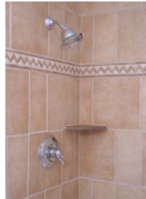
Bathroom Renovation Beautifully tiled shower
