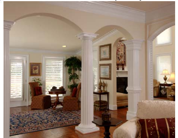
Sunroom Wall Conversion – Arched Cased Opening with Columns
